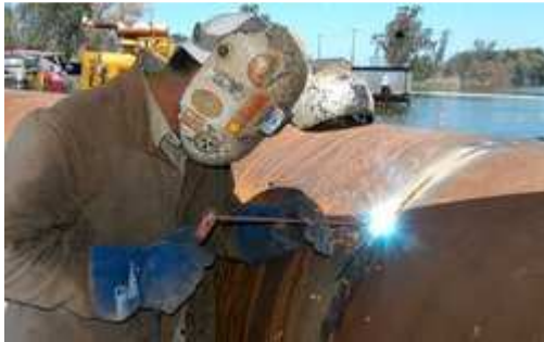
Shielded metal arc welding a pipe
